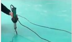
1.1.2 Welded seams must cool to room temperature before trimming in two steps, rough and fine trimming.
